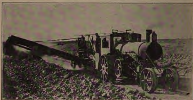
Traction Engine and Elevating Grader Excavating Irrigation Canal.
